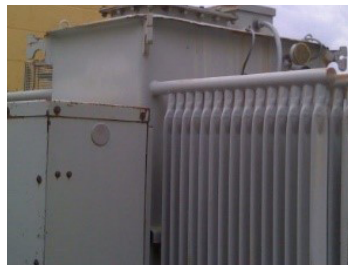
TRANSFORMER RADIATOR — A COMPARISON OF CONVENTIONAL PHOTOGRAPHY AND A THERMAL IMAGE SHOWING THE LACK OF A TEMPERATURE GRADIENT WITH ONLY A DELTA OF 0.6°C BETWEEN SP1 (22.4°C) AND SP2 (21.8°C).
