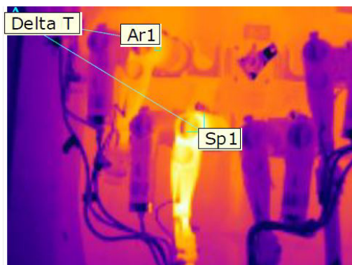
A SIDE BUSHING — A COMPARISON OF CONVENTIONAL PHOTOGRAPHY AND A THERMAL IMAGE SHOWING A DELTA OF 19.3°C BETWEEN SP1 (46.3°C) AND AR1 (27.0°C).
